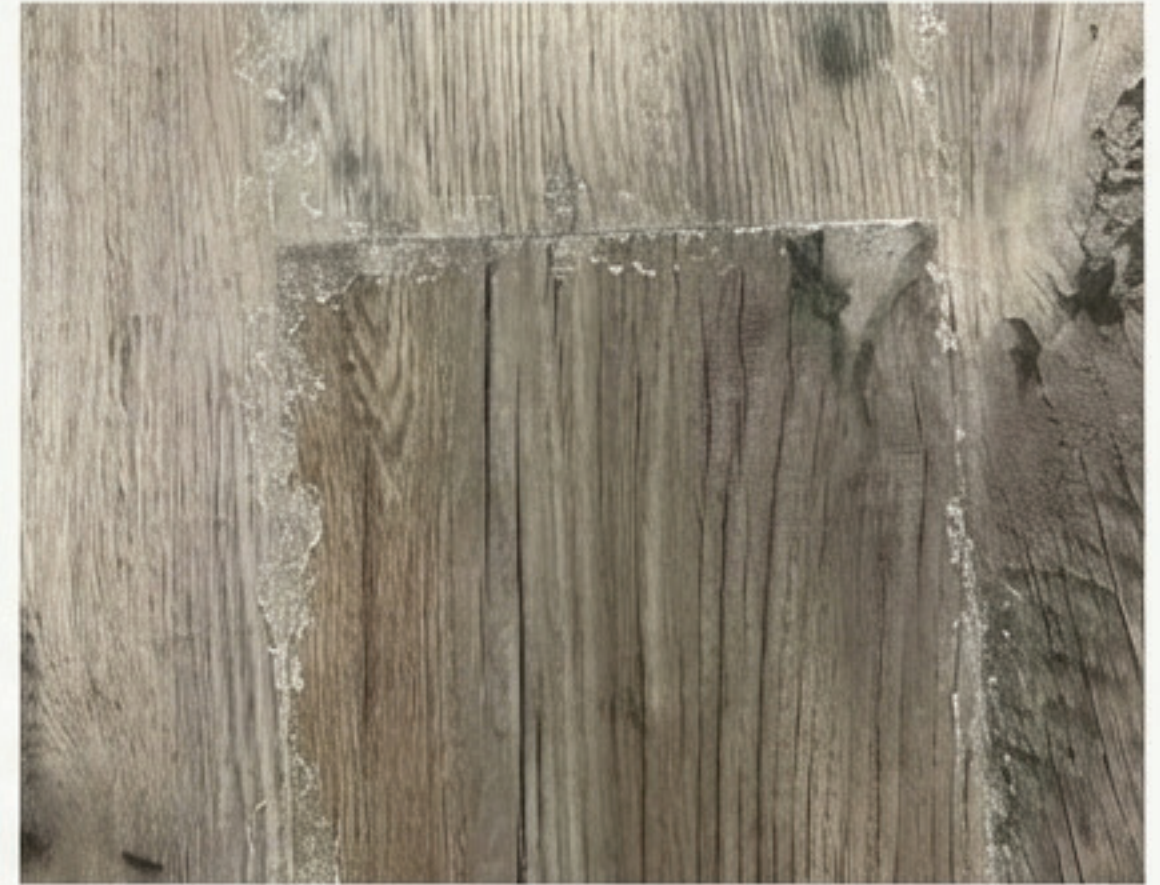
Adhesive Failure
